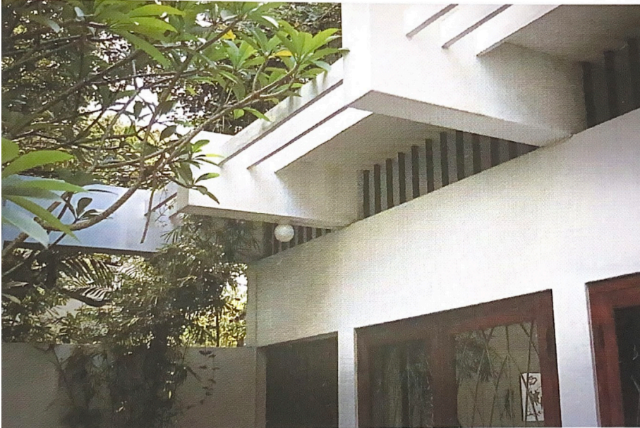
Left: Cantilevering beams and sun breakers on the Kannangara House
